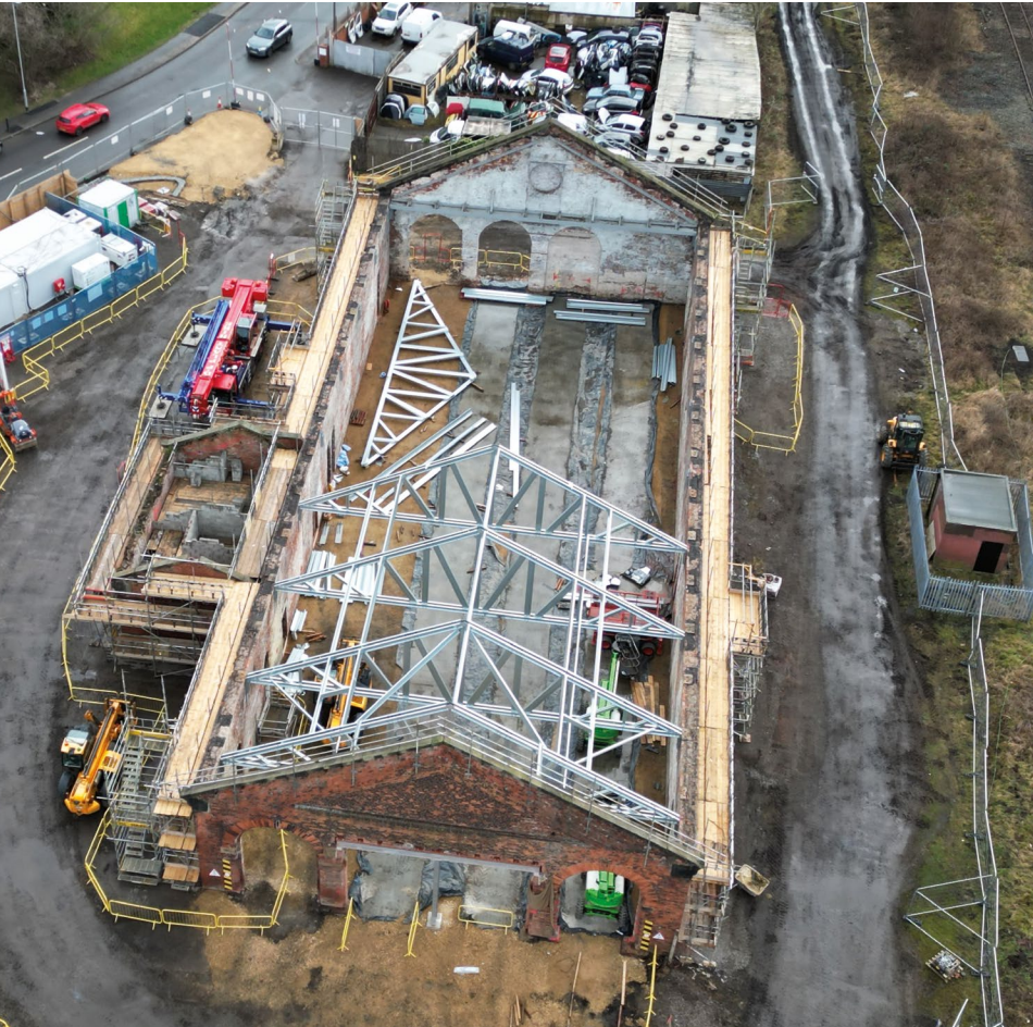
An aerial view of the Whessoe Road engine shed shows the roof trusses being installed.
