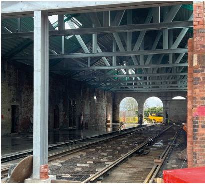
Reinforcing steel mesh in place for the floor to be poured.
