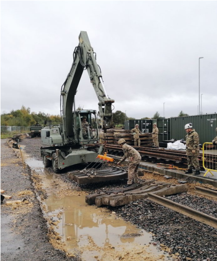
Above: The first concrete sleepers are laid out.
